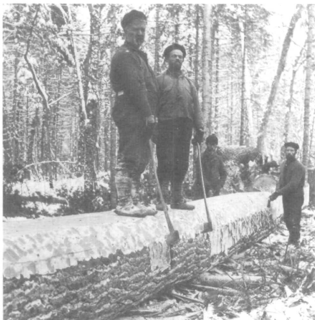
Fig. 7. The scorers moved ahead, notching the timber to the appropriate depth. The hewer followed, using the broad axe to produce a flat surface. (Photo: PAC, neg. no. PA-121800.)
