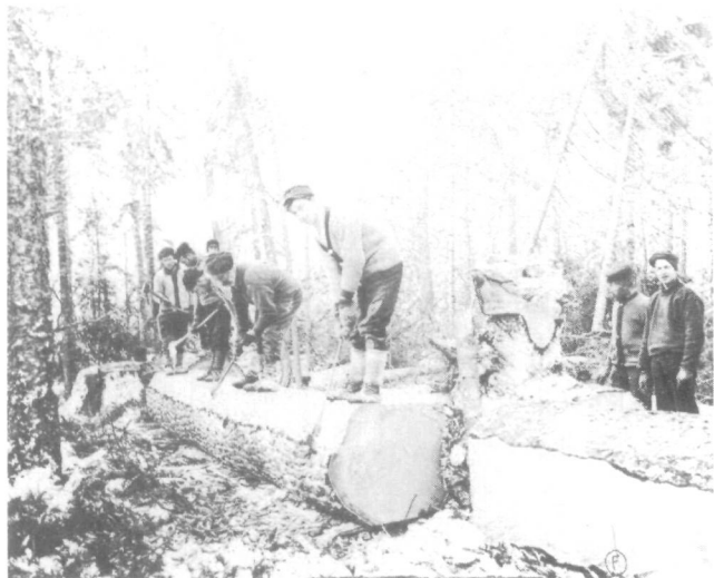
Fig. 5. "Rossing" or removing the bark from a piece of timber in preparation for the chalk line. (Photo: PAC, neg. no. PA-121797.)
