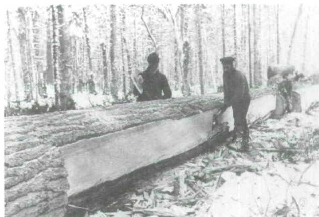
Fig. 4. Hewing square timber. (Photo: PAC, neg. no. PA-121799.)
