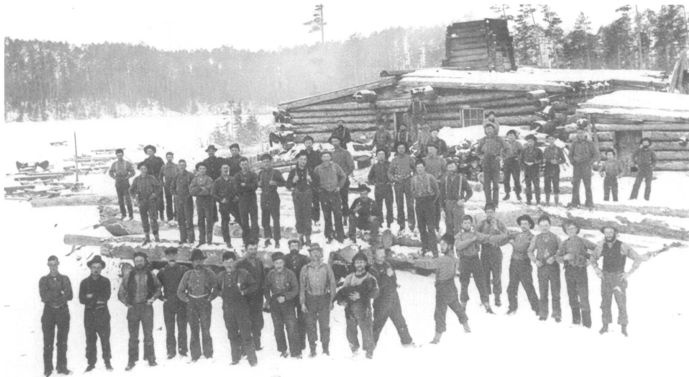
Fig. 2. Booth lumber camp at Aylen Lake, Ontario, ca. 1895. Although taken in the Ottawa River district late in the nineteenth century, this photo illustrates the primitive log shanties built by the larger lumber companies throughout the century. Note the flattened lumber chimney and log construction of both the main shanty in the center of the photograph and the outbuildings. Timber sleighs are to the left. (Photo: Public Archives Canada [PAC], neg. no. C-75264.)
