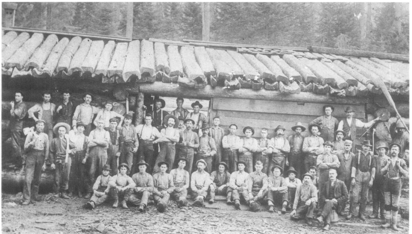
Fig. 3. This lumbering camp, Ontario 1895, illustrates the scoop roof typical of early shanties in Ontario. Note the similarity of dress among the shantymen. (Photo: PAC, neg. no. C-22452.)
